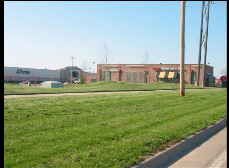
Pedestrian scale building in front of large scale retail
