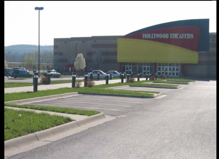
Pedestrian walkways Scaled lighting
